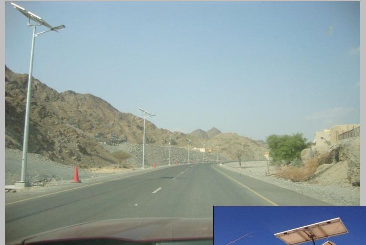
First road with streetlight in Dubai 404 streetlights, 11 KM 2 units 8D-GEL in each post
