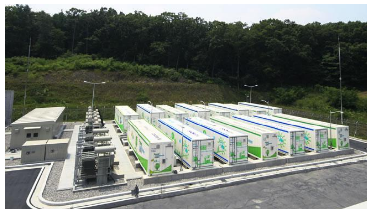
Kokam's 56 MW NMC Energy Storage System
